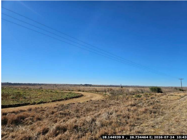
View towards start of 132 kV powerline deviation
