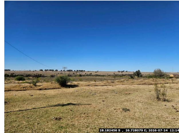
33 kV route towards compressor station
