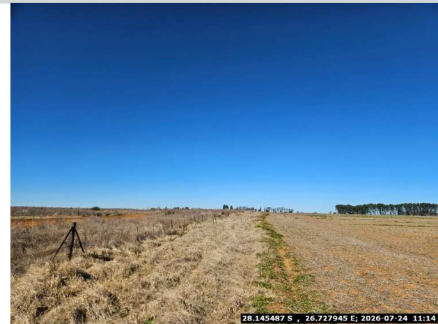
Southward view along the 132 kV deviation route
