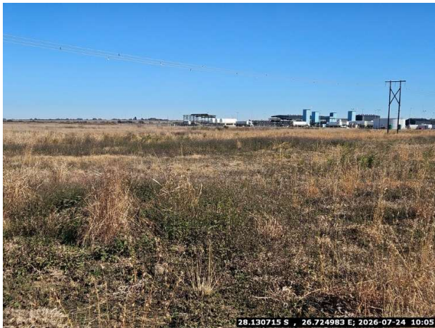
View towards Tetra4 plant where the powerline ends
