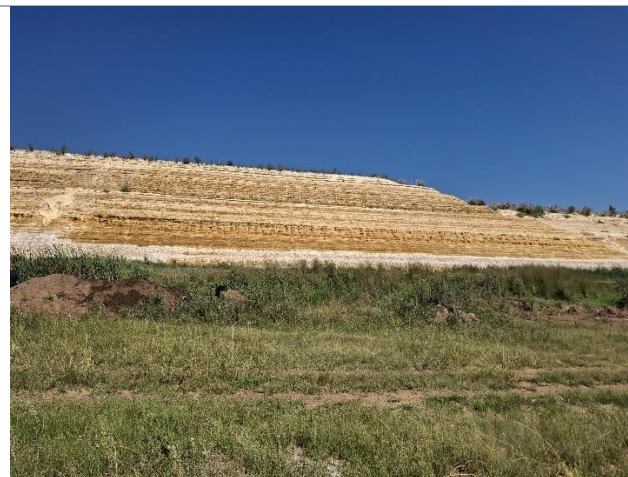
Figure 7: View northeast of the southern side slope of the existing Deelkraal TSF, adjacent to the proposed Deelkraal II TSF.
