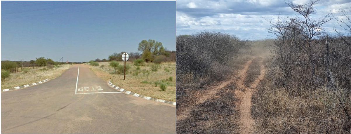
Figure 21: View of the site access road off the R510 (left) and existing local in-field site access to well sites (right).
