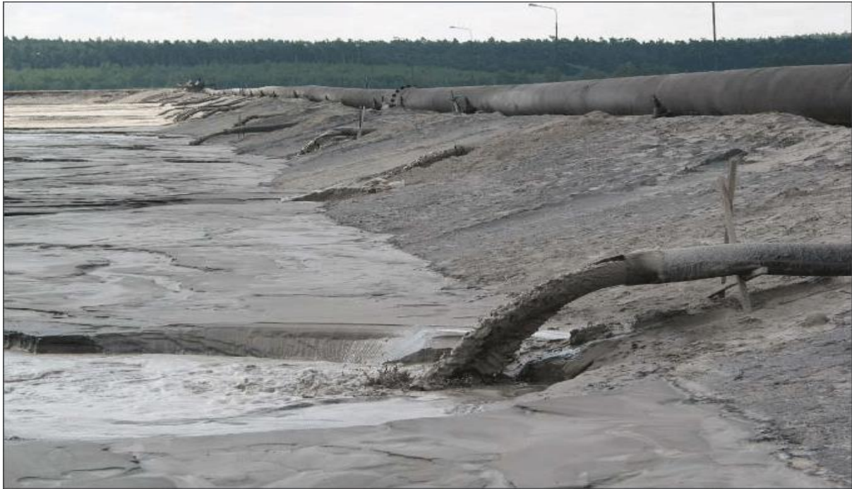
Figure 14: Example of spigot deposition (source: www.researchgate.net )
