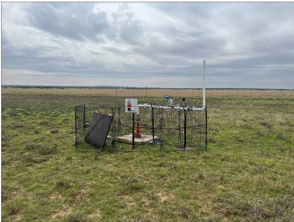
Figure 6: Typical wellhead surface infrastructure (to be connected to underground pipeline if converted to production well).
