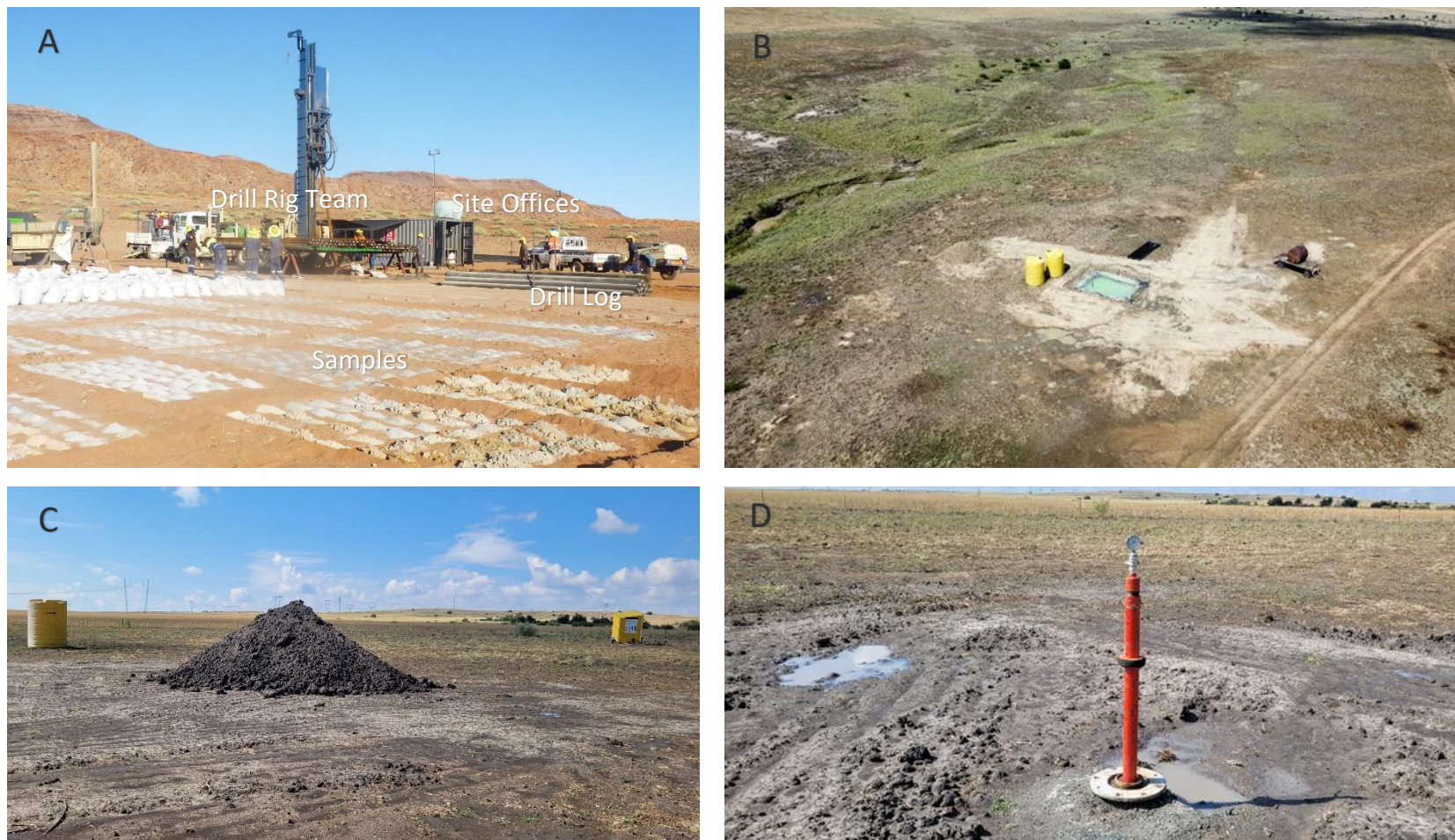
Figure 8: Exploration drilling and potential impacts. (A) Showing the drilling process and associated infrastructure, (B) Showing the drill pad footprint at one of the active Motuoane drilling sites, (C) Showing some of impacts associated with drilling activities including contained vegetation clearance and topsoil heaps and (D) Showing the final exploration well, steel cased and cemented to prevent leaks.
