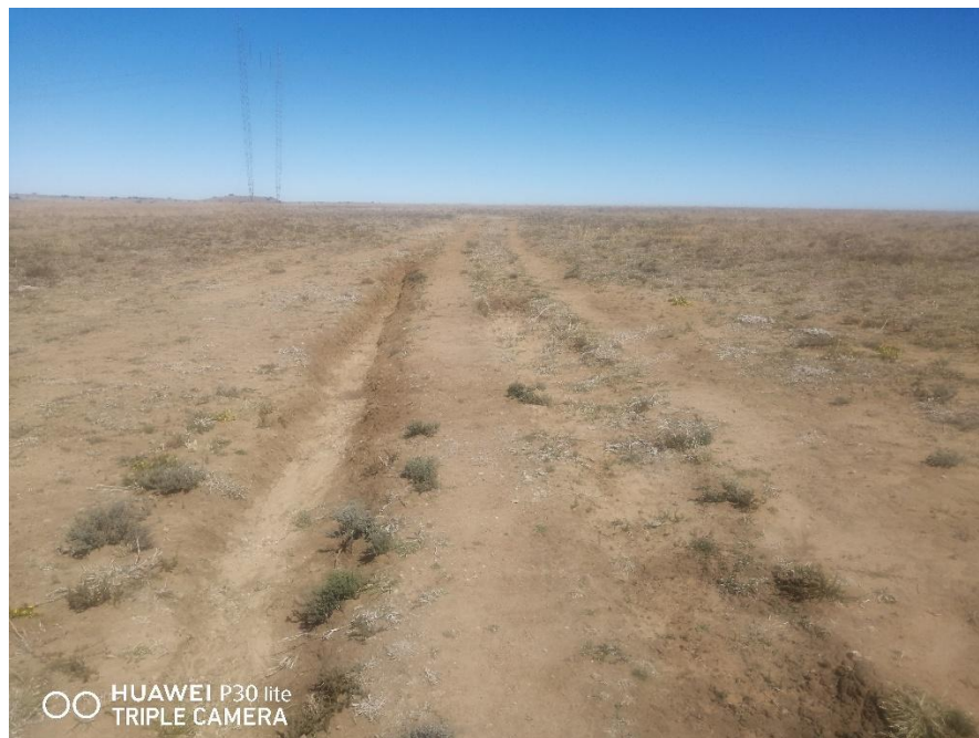
Rill erosion noted on one of the farm access roads within the PR area
