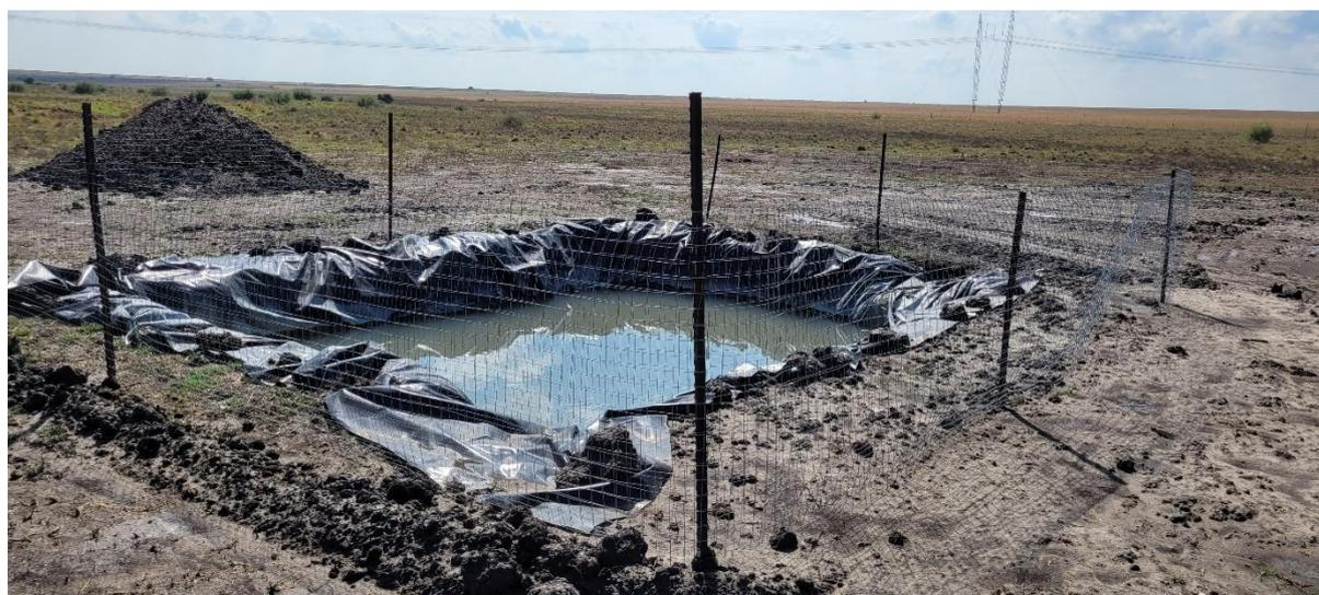
Figure 74: Typical traditional sump pit used for one of the approved Motuoane drilling sites in the region.
