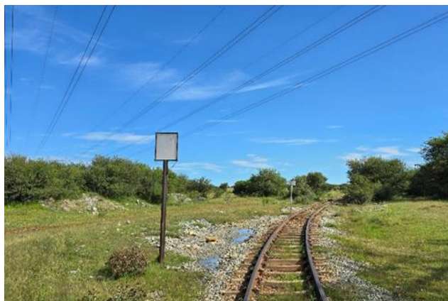
Figure 24: A railway line which appears to be still operational was noted in the western section.
