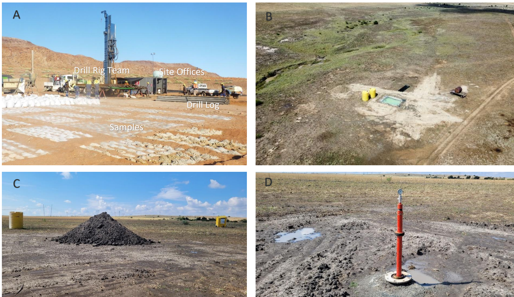
Figure 5: Exploration drilling and potential impacts. (A) Showing the drilling process and associated infrastructure, (B) Showing the drill pad footprint at one of the active D3 Energy drilling sites, (C) Showing some of impacts associated with drilling activities including controlled vegetation clearance and topsoil stockpiles and (D) Showing the final borehole, steel cased and have cemented to prevent leaks.
