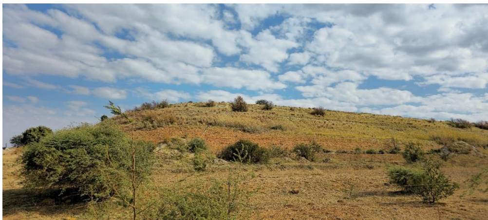
Figure 39: Steep embankment of the Mponeng Lower TSF with alien vegetation and maintained gravel access road.
