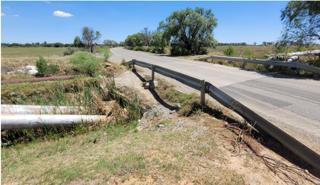
Figure 9 Example of a typical Harmony pipeline culvert proposed for the project at the road crossing
