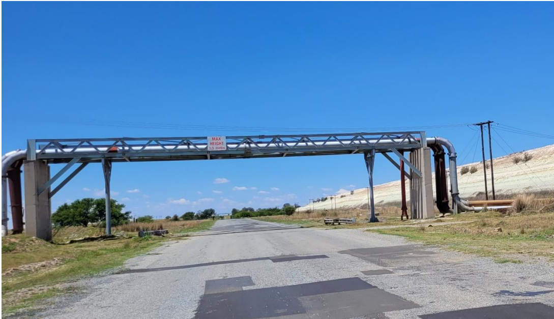
Figure 8: Example of a typical Harmony pipeline bridge proposed for the project at the water crossing
