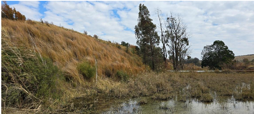
Figure 43: Northern boundary of the Mponeng Lower TSF showing the steep embankment and vegetation including alien invasive trees and a potential wetland.
