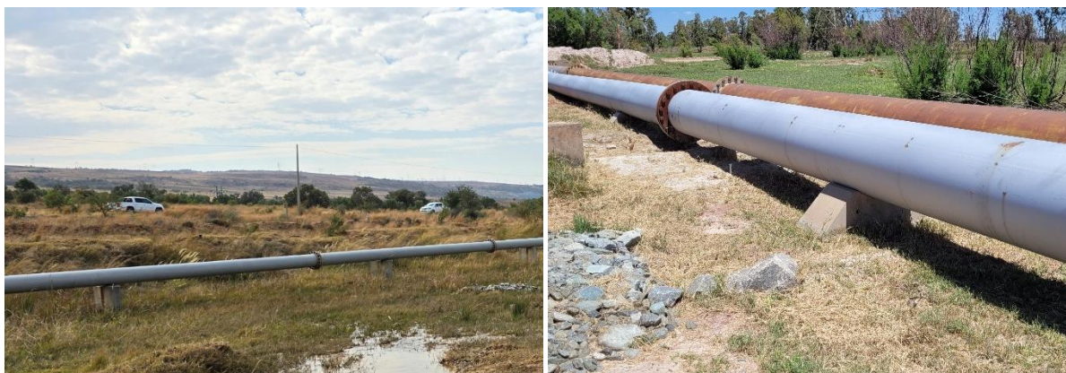
Figure 7: View existing aboveground residue deposition pipeline on site (left) and view of typical slurry and return water pipes taken from a different Harmony plant (right)
