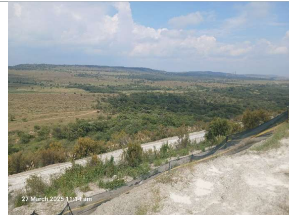
Figure 13: View from the road on the TSFs to the south of the study area towards the west. The netting for dust mitigation is visible in the foreground on the side slopes and the existing plantation for phytoremediation in the background.
