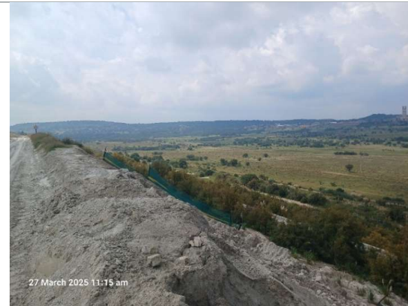
Figure 15: View from the road on the TSFs to the south of the study area towards the east. The netting for dust mitigation is visible in the foreground on the side slopes of the TSFs.
