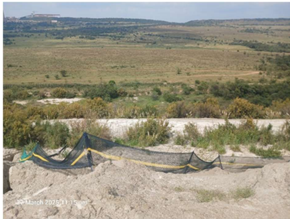
Figure 14: View from the road on the TSFs to the south of the study area towards the south. The netting for dust mitigation is visible in the foreground on the side slopes of the TSFs.
