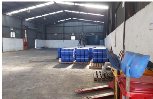
Figure 12: Bunded warehouse with chemicals stored in containers.
