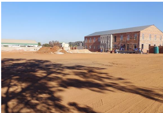
Figure 11: Administration building under construction.
