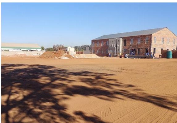
Figure 11: Administration building under construction
