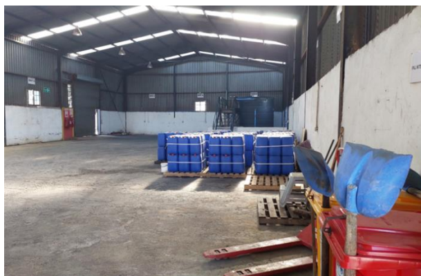
Figure 12: Bunded warehouse with chemicals stored in containers
