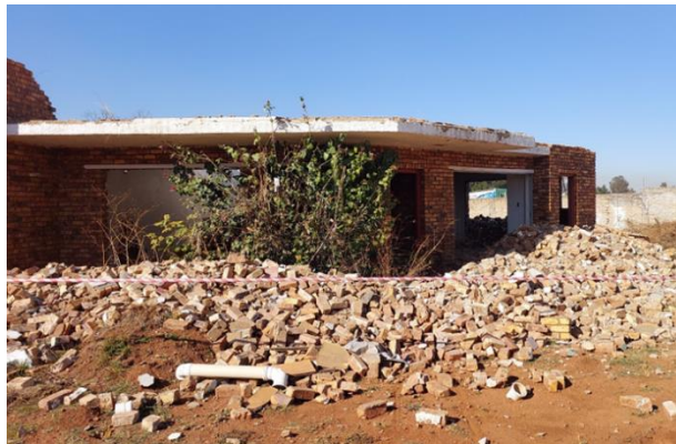
Figure 10: Dilapidated buildings to be demolished
