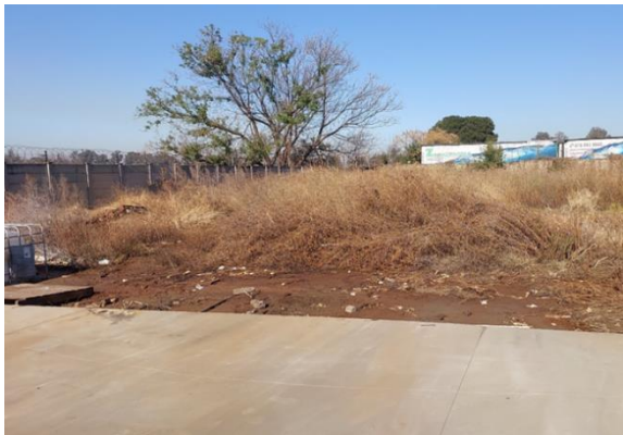
Figure 9: Disturbed vegetation on site
