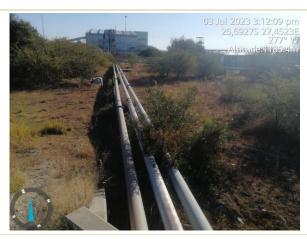
A view of existing pipelines running between K3 shaft and K3 concentrator plant placed on concrete plinths. The pipelines cross the road via concrete culverts. Shrubs were noted on site.
