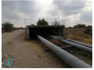
North view along the existing K4 return water tie in and K4 return water dam. The new proposed pipeline is to be placed along existing pipelines through the existing culvert across the drainage line towards the K4 return water dam.
