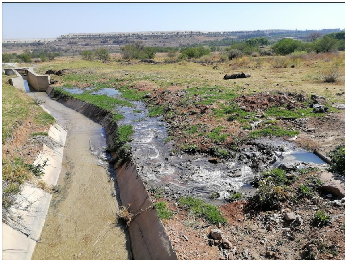
Figure 19: Manhole Leak at Site Golf 2
