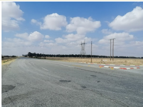
SW – Theseus Oryx 132 kV Powerline.
