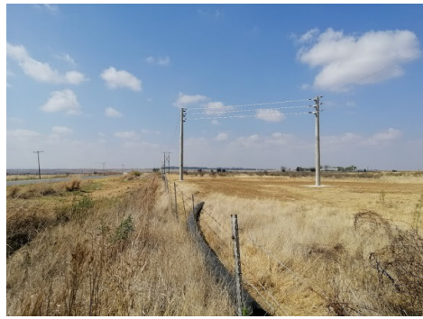
SW – Existing powerline pylon
