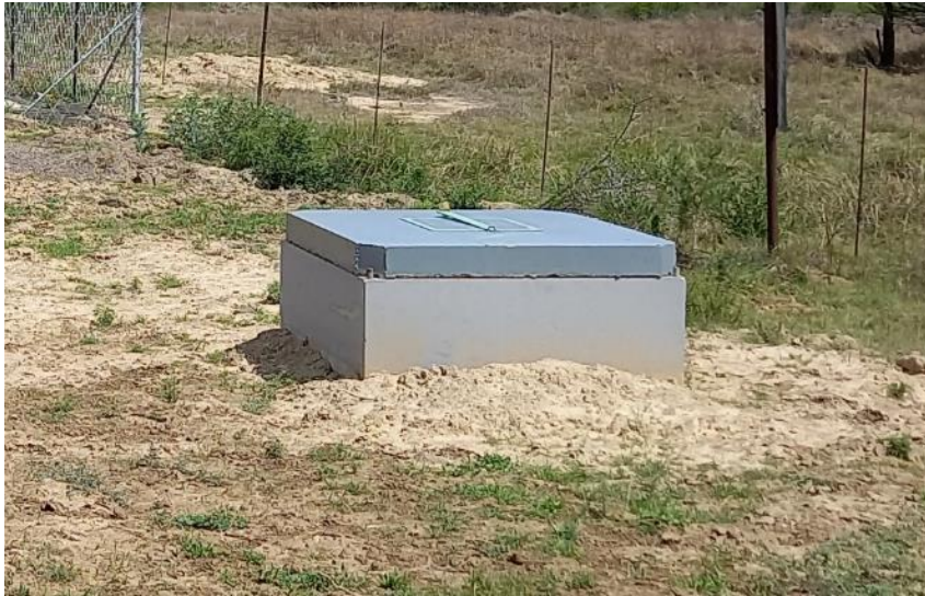
Figure 10: View of an existing low point drain constructed as part of Cluster 1.
