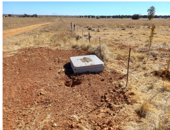
Figure 12: Low point drain.
