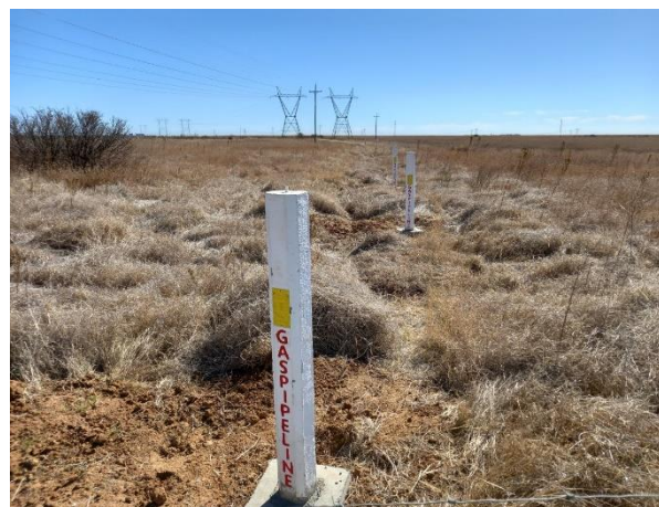
Figure 14: Rehabilitated pipeline route.
