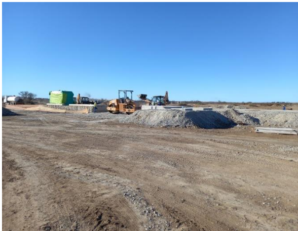
Figure 17: Typical example of helium / LNG Plant construction.
