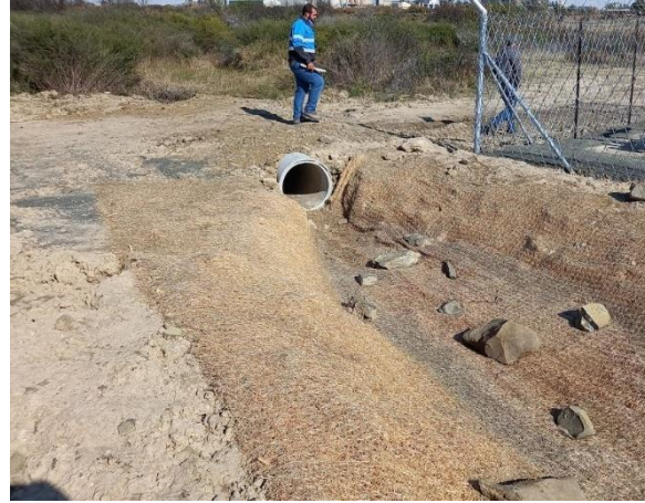
Figure 16: Typical example of access road flume pipe.
