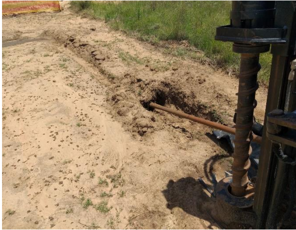
Figure 9: Typical example of exploration drilling.
