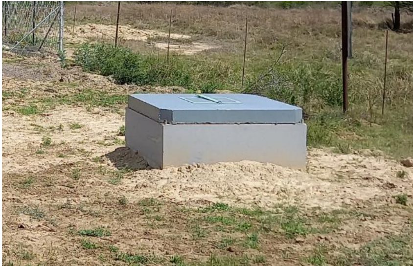
Figure 5: View of an existing low point drain constructed as part of Cluster 1.
