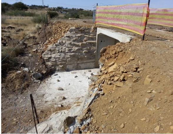
Figure 15: Typical example of culvert on access road.
