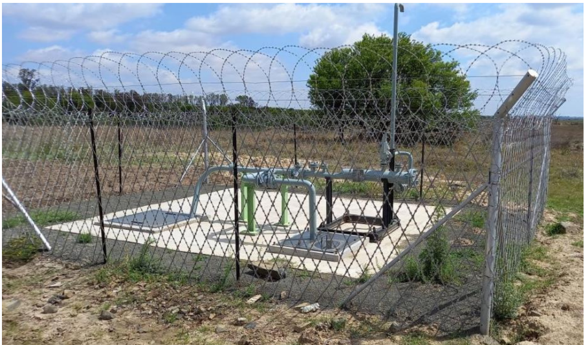
Figure 4: View of an existing pigging station constructed as part of Cluster 1.
