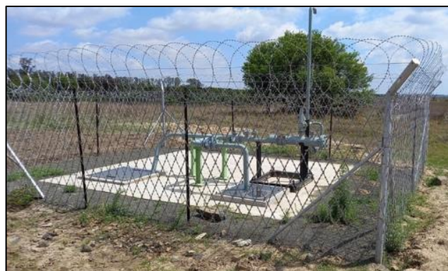
Figure 7 - View of an existing pigging station constructed as part of Cluster 1.
