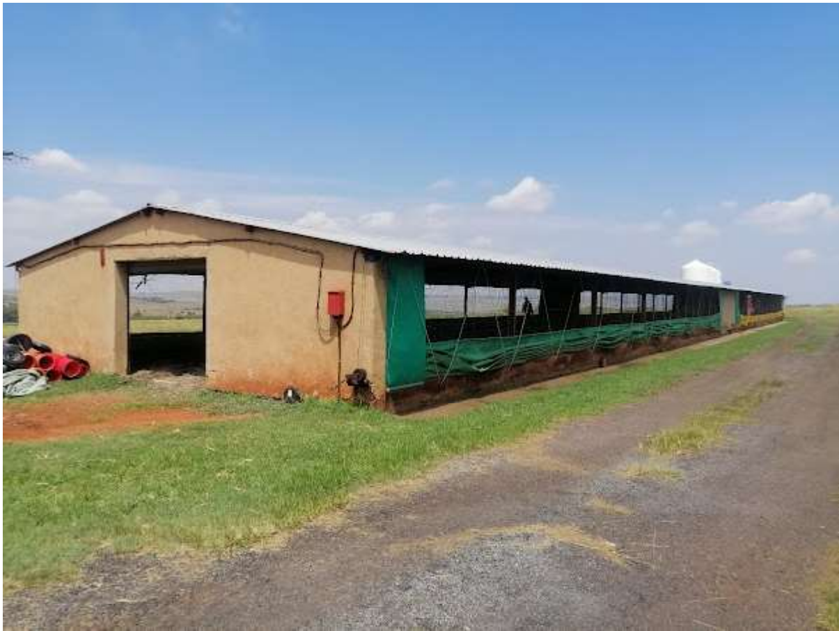
View of the existing poultry house
