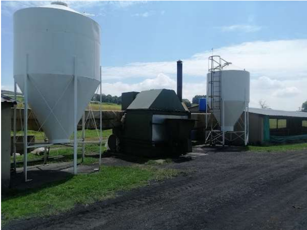
Existing food silos and boilers
